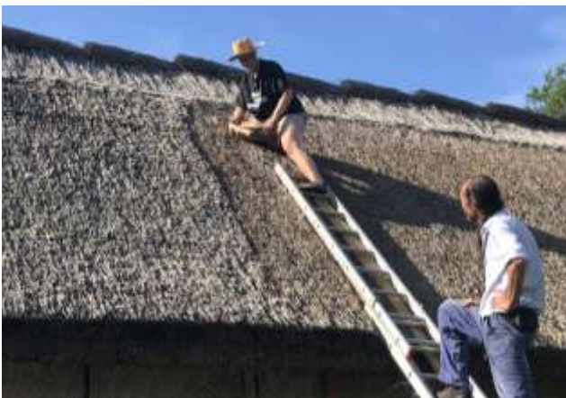
Work on a thatched roof: another part of the effort behind the farm.
